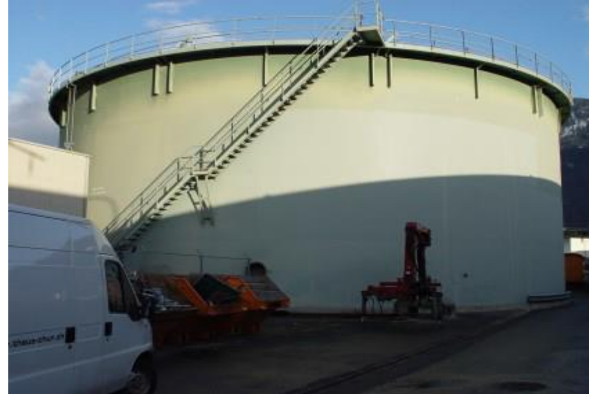
Tank, anti-corrosion coating
