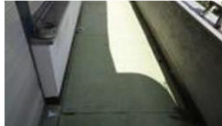
Paint and sealants on balconies
