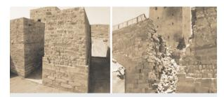
Marid Old Dam before and after image. Photo credit: Hussain Bukhaiti. Satellite imagery collected on 29 October 2015 shows one of the retention towers severly damaged with visible debris in the middle section of the Southern Dam sluice.
